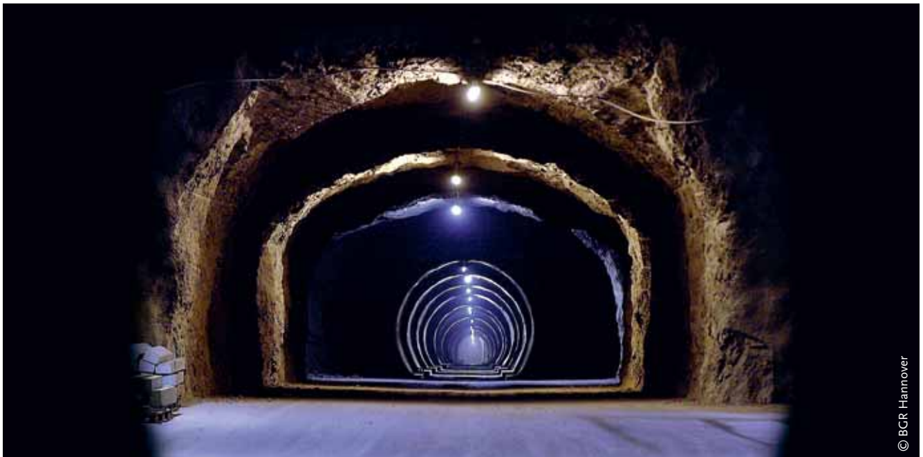
FIGURE 1: Exploration tunnel in the international Mont Terri Rock Laboratory (Switzerland). For about 20 years, scientists carry out experiments on the long-time safety of repositories in Opalinus Clay (sedimentary rock).
